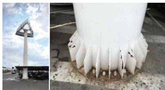
Figure 8(ab). Tall metallic pillar, retained in its base by screws. Note the heavy reinforcement with metallic flanges at the base to counter the lateral forces from all directions.
